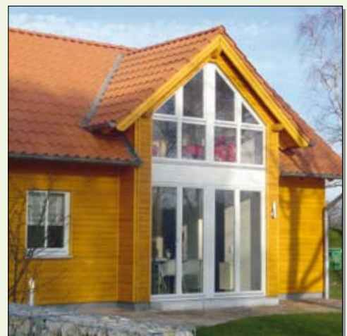
Timber cladding treated with Osmo Park Lane 7265 Light Ochre transparent
