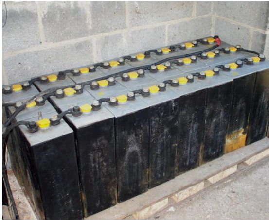
24 x 600 amp-hour, 2-volt cells wired in series
