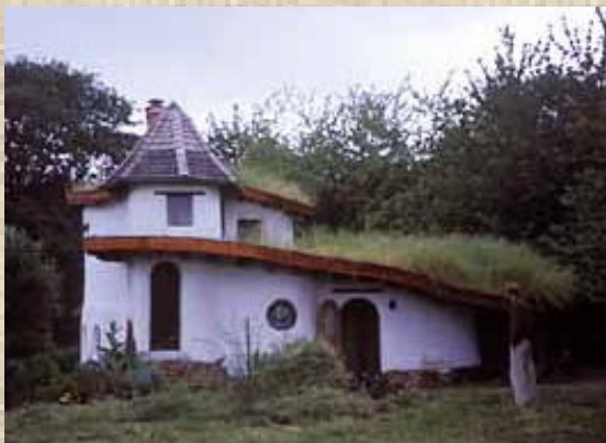
a modern cob home with living roof, in the US
