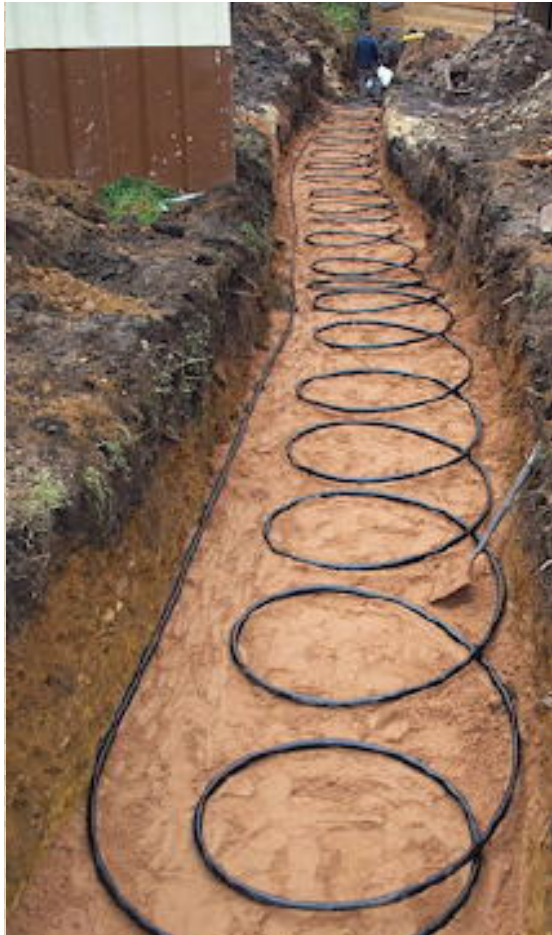
the ground loop collector pipe is laid in a trench
