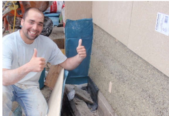
removing the shuttering to expose a raw hempcrete wall
