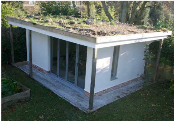
a hempcrete garden office with a living roof
