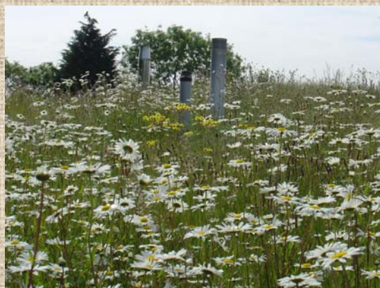
not a flower meadow, but our course tutor John's roof 10 years after installation, during which time he's done precisely nothing to it; you can tell it's a roof from the flue pipes!
