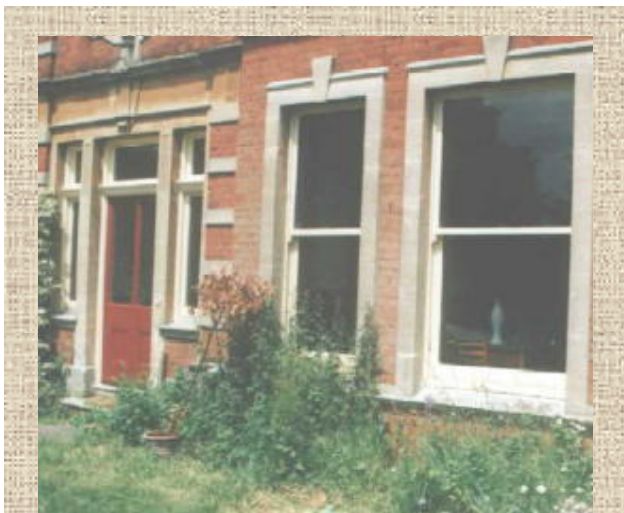
eco-paints on doors and sash windows: Redfield has changed from waterproof paint to eco-paints on all 200 windows on the house and stable block; only natural, breathable materials are now used – for example lime mortars and linseed oil putty instead of cement mortars or mastics.
