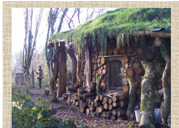
when it comes to building a home on a smallholding, you can go super-eco, like this off-grid roundhouse with turf roof on a smallholding in Pembrokeshire.
