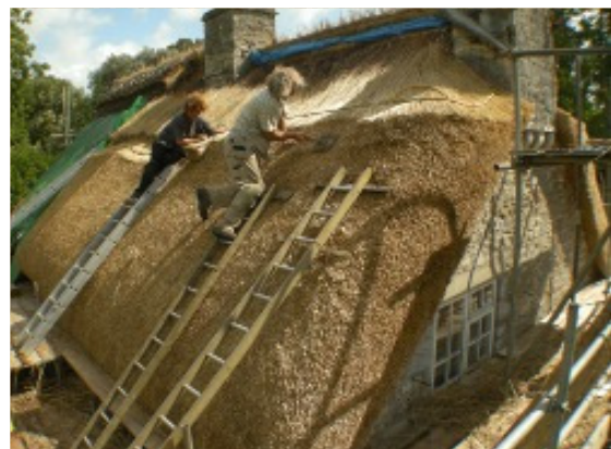
thatchers at work on a roof
