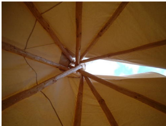
looking up through the smoke flaps that allow the smoke from the fire to escape.
