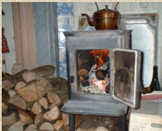
a basic wood stove sitting on a slate base, with a flue at the rear, passing through a metal plate to the chimney; seasoned wood is stacked next to the fire to dry further.
