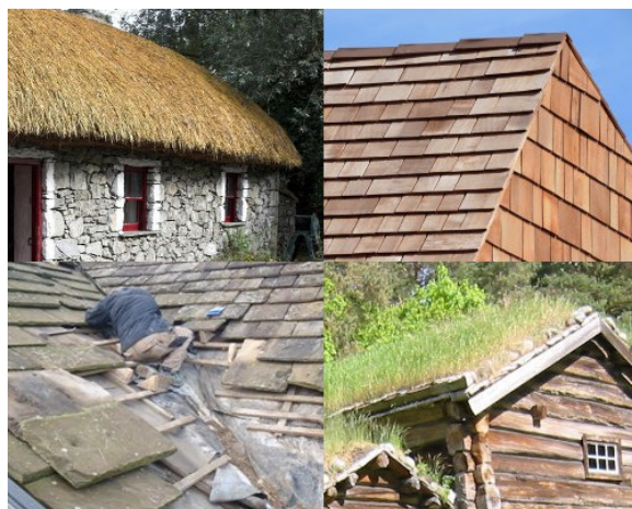
Natural roofing materials (clockwise from top left): thatch; wooden shingles; turf; stone.
