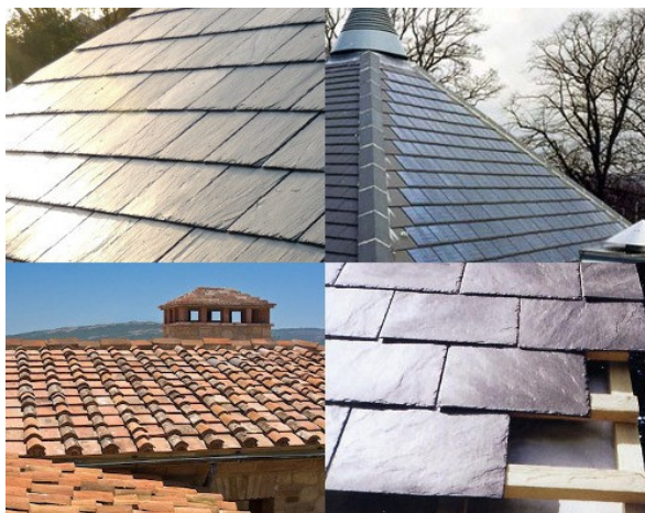
Slates & tiles (clockwise from top left): natural slates; solar tiles; recycled plastic slates; clay tiles. All involve less embodied energy and pollution than concrete tiles, and of course the solar tiles generate electricity.
