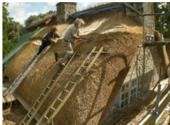
Thatchers at work on a roof.
