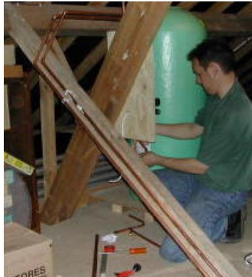
*installing a twin-coil cylinder with pump & control set (for solar hot water) in a loft, with copper pipework and 45° elbows*
