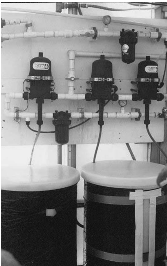
Figure 4.5 Dosers (injectors) for dispensing stock solutions are shown in place over stock solution barrels. Dosers are adjustable so that they can deliver a specific aliquot of stock nutrient solution into a flow of water for constituting a nutrient solution for delivery to plants. One doser is used for each stock nutrient solution.
