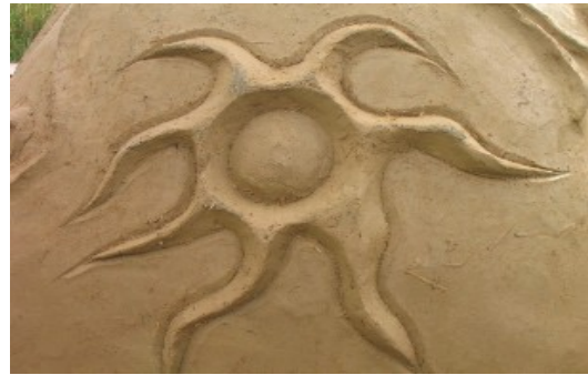
Plastering details added to the final, sieved layer.
