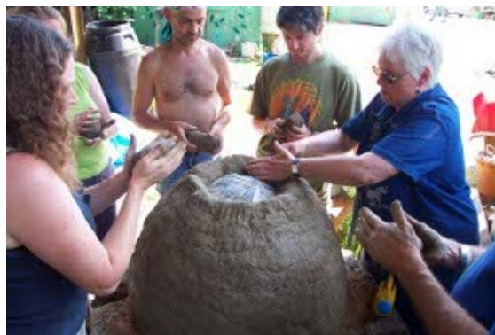
Building up an oven around a dome of sand.
