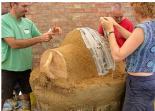
Covering a dome of damp sand (with wooden door attached) with wet newspaper; the oven will be built around this, and then the sand scraped out to form the chamber.
