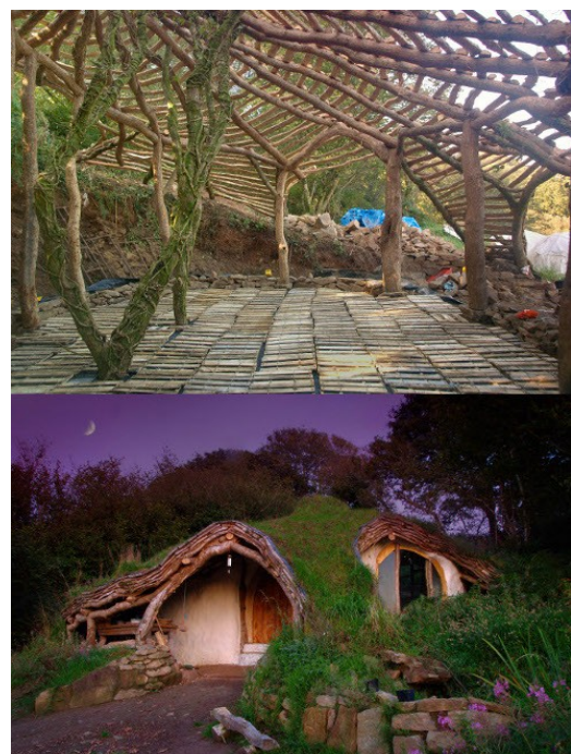
Frame for earth-sheltered house and finished house; cost, £3000; pic: Simon Dale.
