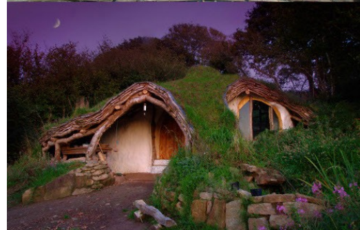
Frame for earth-sheltered house and finished house; cost, £3000; pic: Simon Dale.
