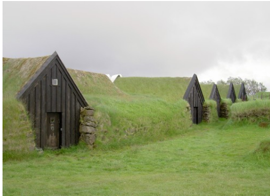
Earth-sheltered houses at Keldur in Iceland.
