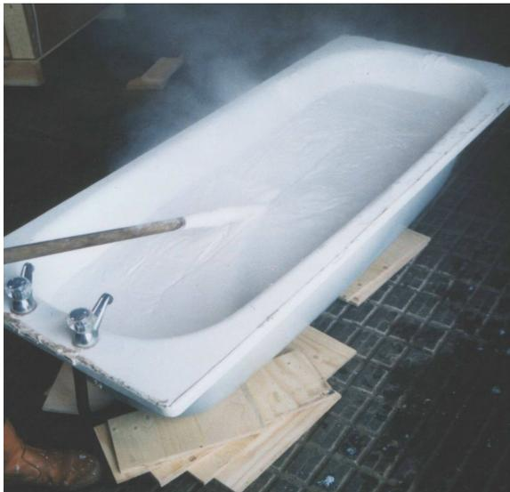
*Quicklime being slaked in an old bath: the lime is added to the water, not water to lime, as it could cause an explosion. The ratio of water:lime is 3:1. To ensure that all the lime is slaked, rake the mixture for 10 minutes. There's a violent reaction, and heat and steam is given off. When cool, the lime putty can be stored in plastic buckets indefinitely as long as there's a layer of water on top.*
