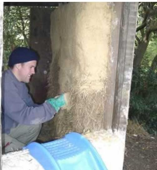
*Lime rendering a straw-bale play-house: one part lime putty is mixed with 3 parts sharp sand. The walls are sprayed with water first; apply two coats, and allow each to dry slowly by covering with wet sacking.*
