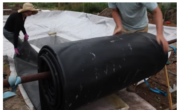
Unrolling the pool's EPDM liner.
