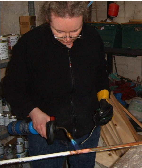
Soldering two lengths of copper pipe together using a straight connector.
