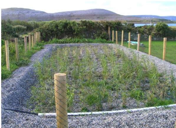
Newly planted domestic gravel reed bed system for septic tank effluent treatment prior to percolation.
