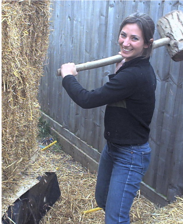
A 'persuader': another home-made tool, this time for gently persuading bales into the position you want.
