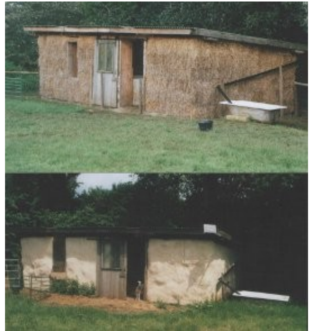
Redfield Community's straw-bale sheep shed before and after lime rendering.
