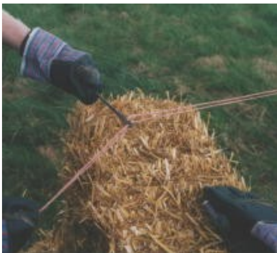
Baling needle: this home-made tool allows you to cut and re-bind bales to any size necessary to fit a gap or a corner.
