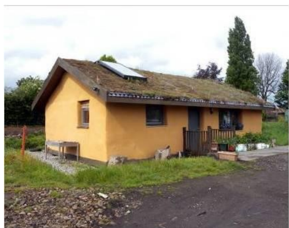
Lime-rendered straw-bale cottage with living roof.
