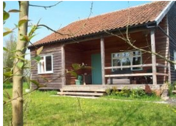
This stud frame house has timber cladding, but conventional roofing tiles; an alternative is wooden roofing shingles, which you can buy or make yourself. You can just make out at the base of the house on the right, that it's sitting on brick pillars.
