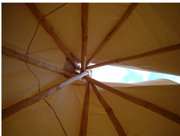
Looking up through the smoke flaps that allow the smoke from the fire to escape.
