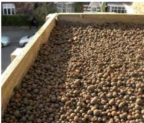
Well-drained substrate. Dusty Gedge/Livingroofs.org
