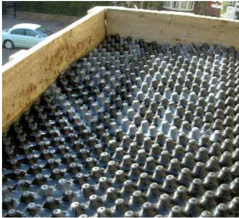
Drainage layer. Dusty Gedge/Livingroofs.org
