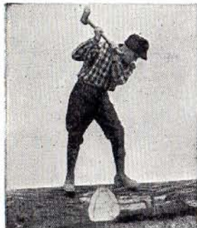
Fig. 23.—Top position for Backhand Stroke, bringing axe into line with other face of V-shaped cut.
